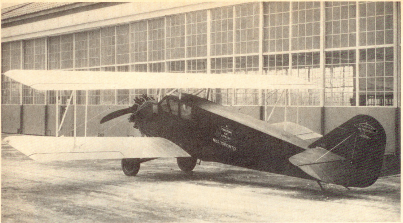
The production SB-1 Detroit had a redesigned fuselage with cleaner lines and greater depth, but retained the classic gap between the top of the fuselage and the bottom of the upper wing. Ford Motor Co. photo.
